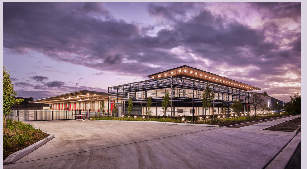
Office and Warehouse facilities with 43 car spaces
